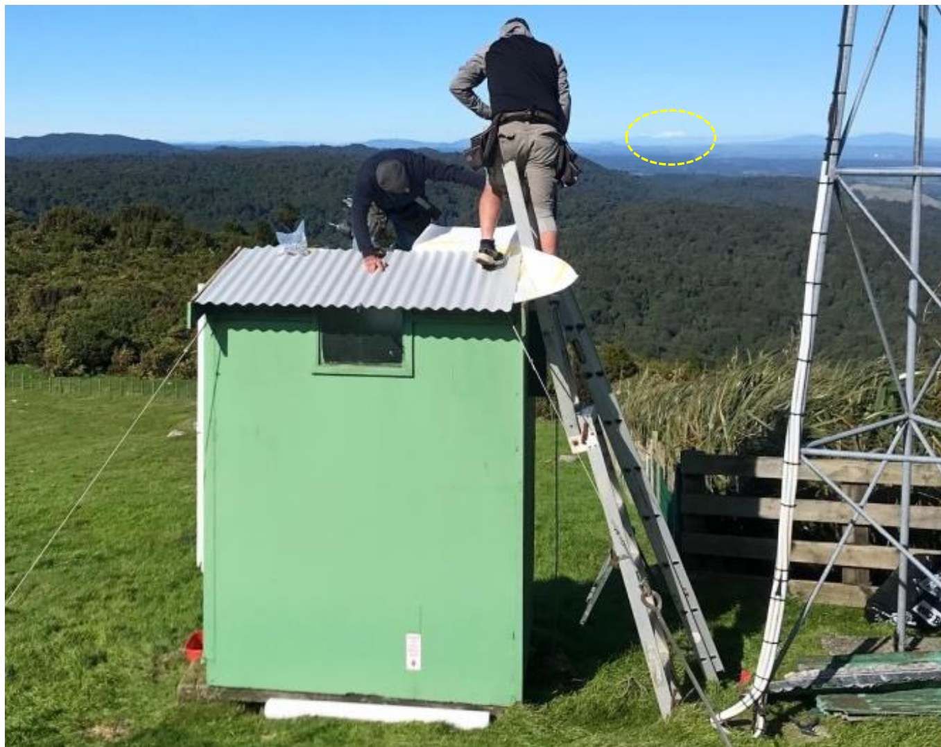
Contractors installing our new ColourSteel roofing iron over (white) synthetic underlay. Observe snow visible on Mt Ruapehu 159km away (circled) to left of the tower.
