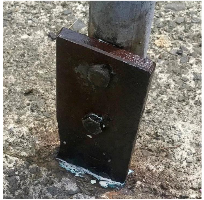
South tower footing following first treatment, March 2026, Rust Converter having darkened the steel.
